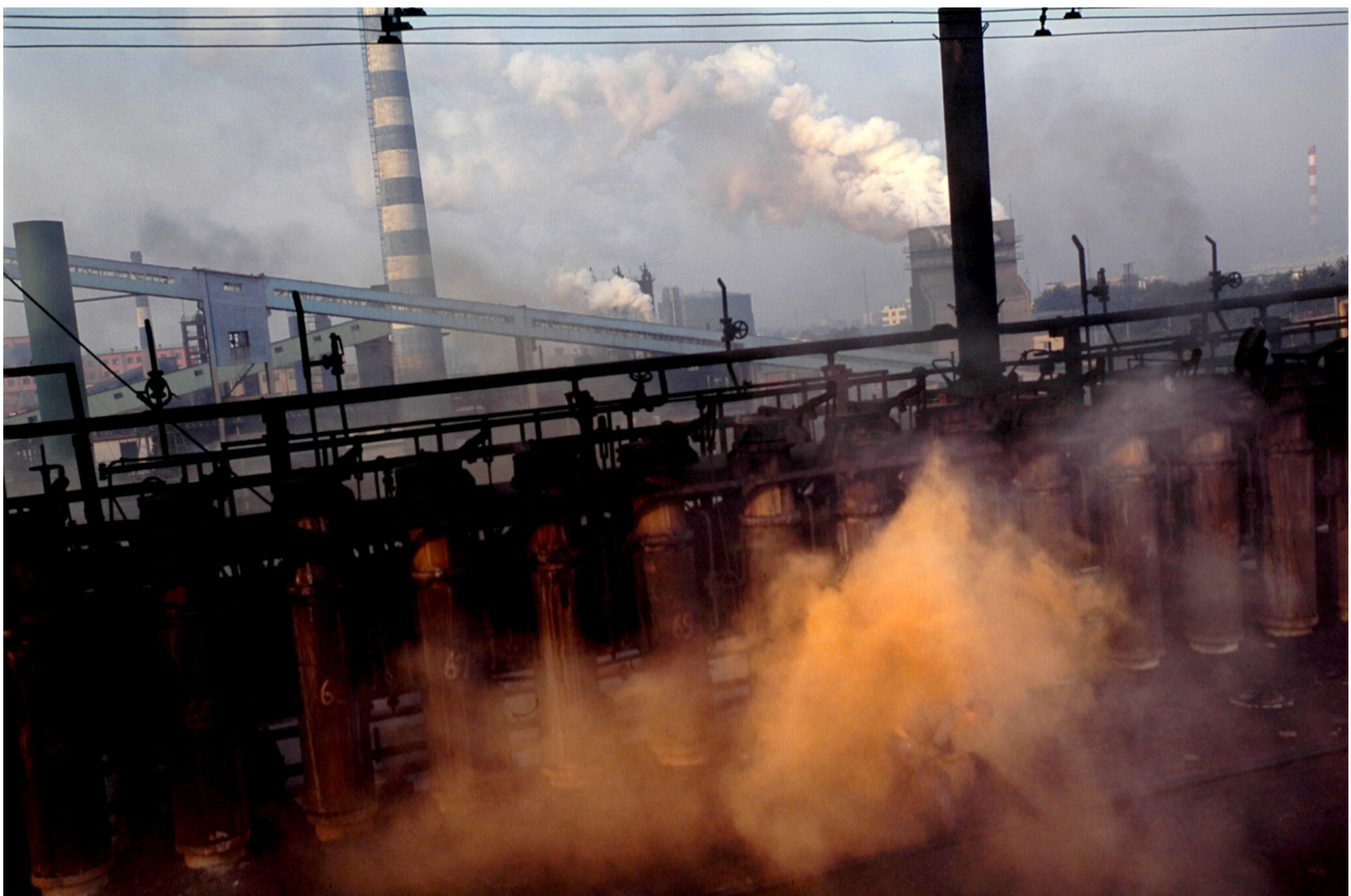
Clouds of toxic yellow smoke are emitted when the pressure inside the furnace is too high, at Tianhong Coking Plant, Henan province, in 2006 ( Niu Guozheng )
