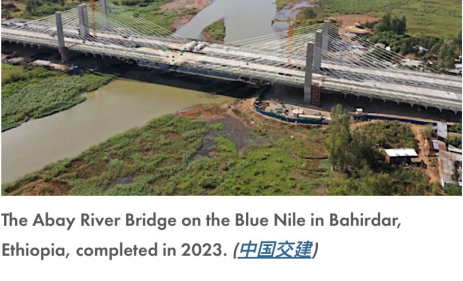
The Abay River Bridge on the Blue Nile in Bahirdar, Ethiopia, completed in 2023. (中国交通)
